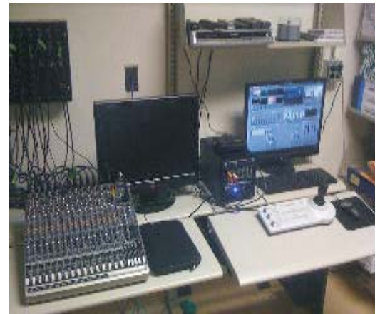
Above: New control room at the library.
